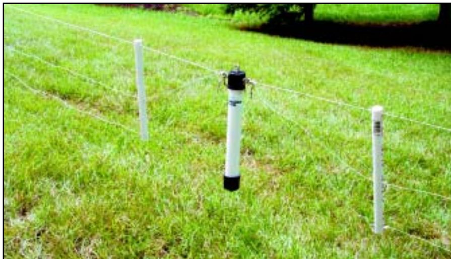
Figure 7—Close-up of the center insulator/balun of a tri-band N4GG Array. Note that all support of the lower wires is provided by the uppermost wires.
